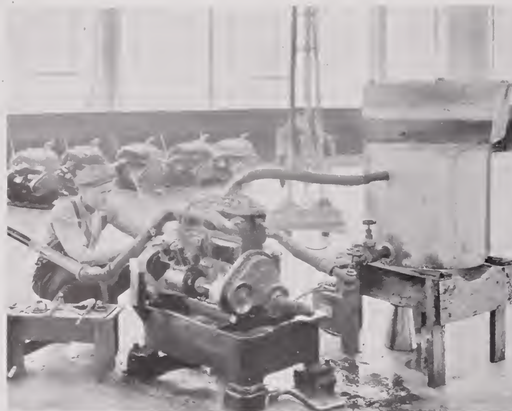
BLOCK-TESTING MODEL 250 MOTORS
